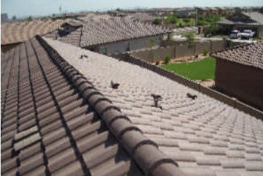
Cement tile roof
