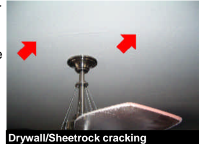
Drywall/Sheetrock cracking
